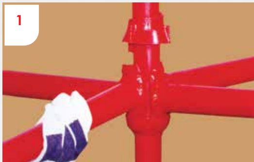
1 Fix ledger blade ends into lower cup
