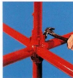
Tighten with a hammer blow
